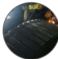
In-Situ Welding of Buttons in Sintercast Liners
